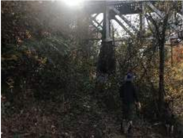
Approaching Trestle on South side
