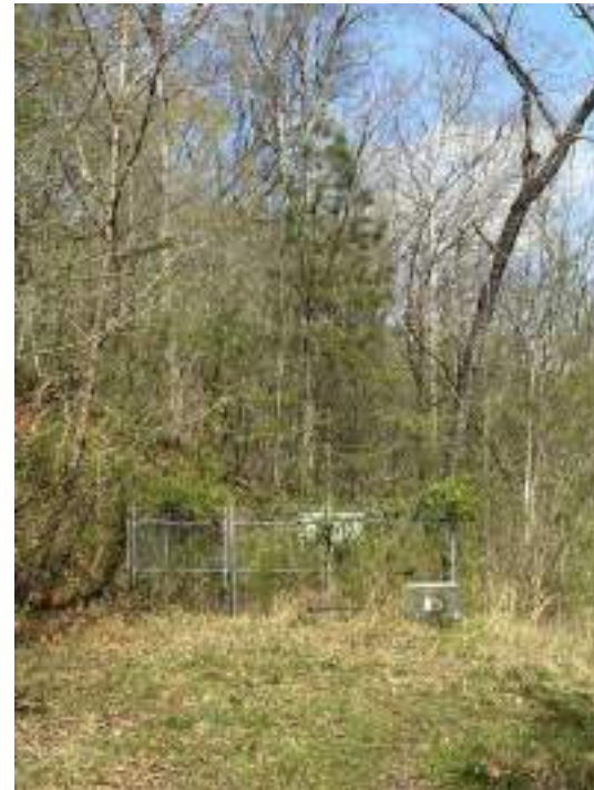
Existing Substation Enclosure
