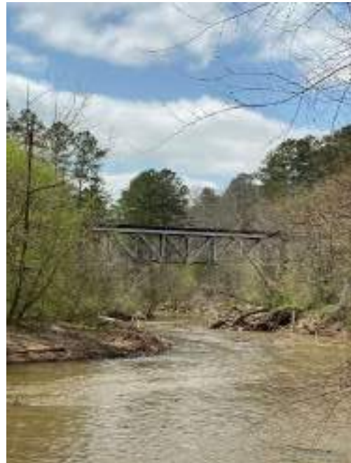
Approaching Trestle on North side
