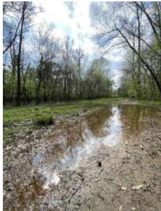
Wet Area on Sewer Easement
