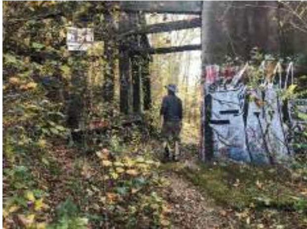
Trestle on South side
