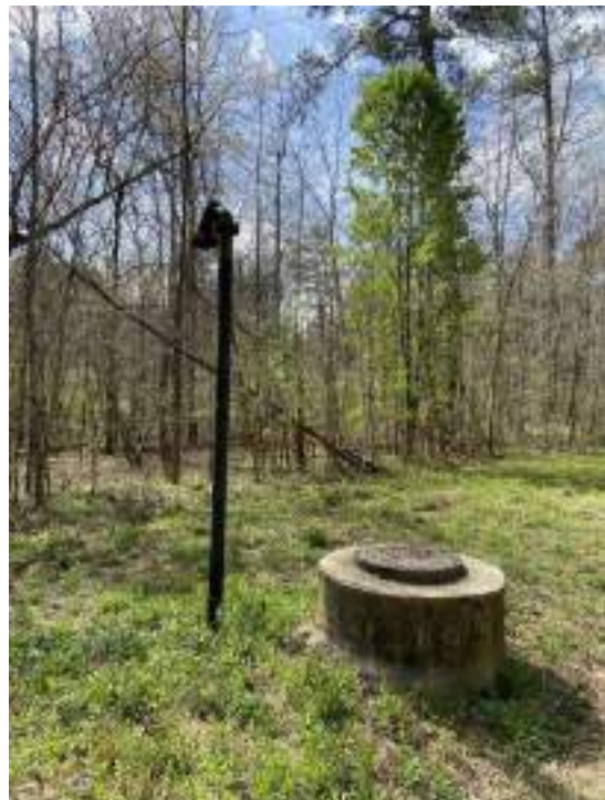
Manhole along Existing Sewer Easement
