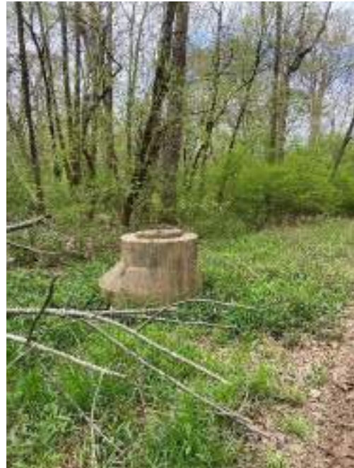
Sewer Line Crossing the River on North Side
