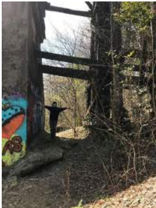
Trestle Bridge Clearance
