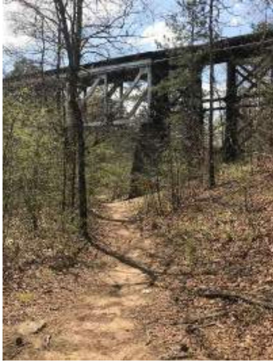
Approaching Trestle on north side
