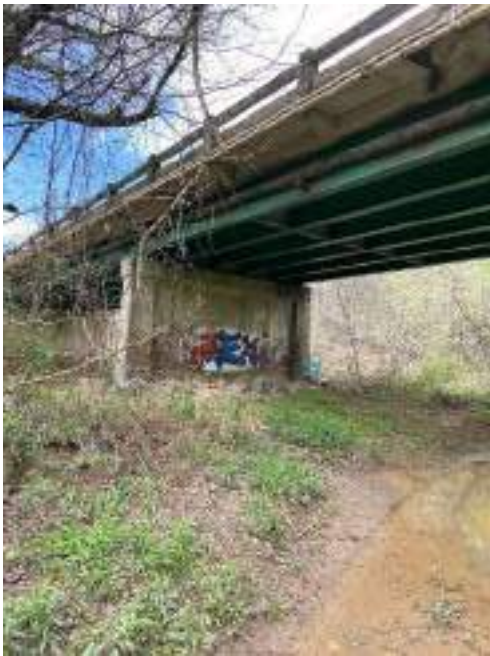
Highway Bridge on North Side
